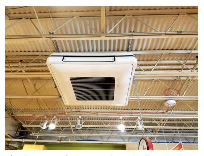
The Daikin VRV (Variable Refrigerant Volume) heat pump system is about 40 percent more efficient overall than a conventional heat pump system. Case studies have shown the system to be 60 percent more efficient while cooling in the summer. The system also allows for "free cooling" using outside air during moderate weather, such as in the fall and spring, further reducing energy use.
